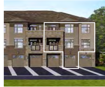
REAR, Interior Unit
