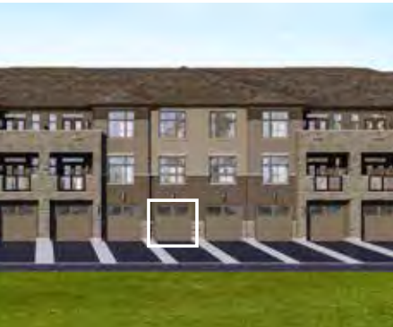
REAR, Interior Unit
